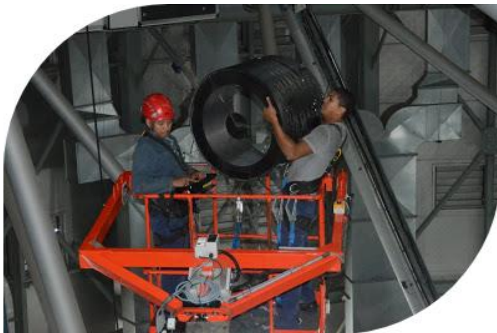
Above: Nicolaas Jacobs and Timothy Fransman removing the lower section of the SAC baffle.
